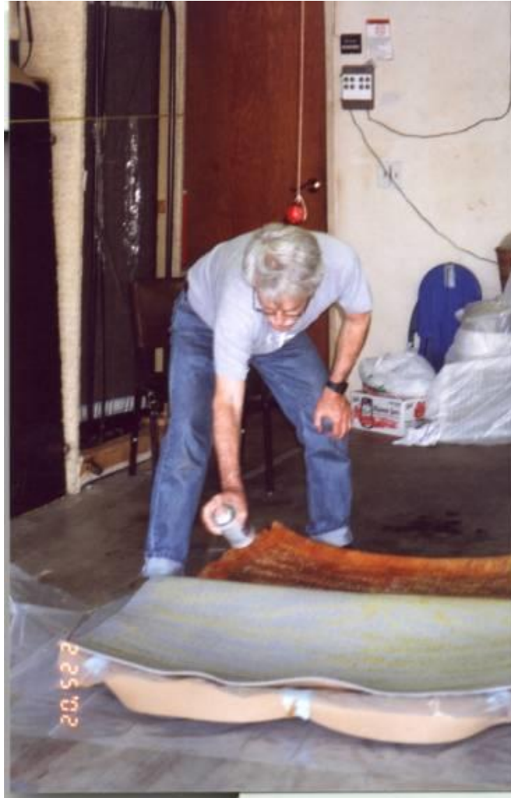
Figure 5. Applying adhesive.
