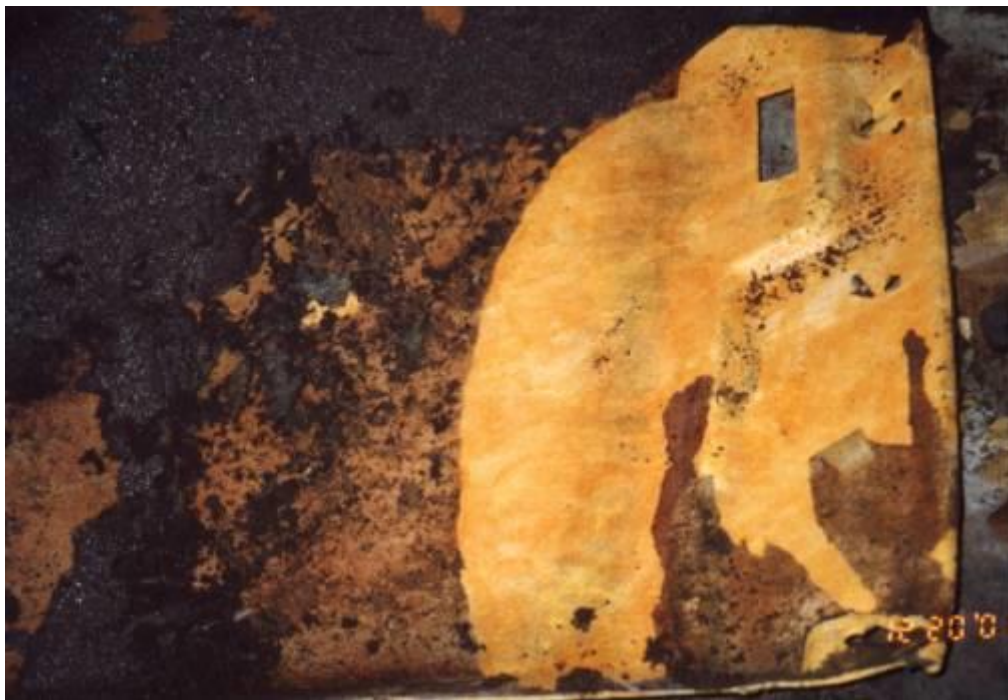
Figure 2. Stripping paper membrane from shell (not necessarily recommended)
